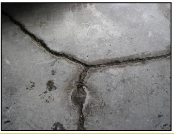
These cracks patched with polyurethane sealant then painted over with a concrete and Lucite mix.
